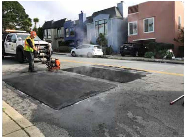
Installing Speed Cushions on Teresita Blvd
