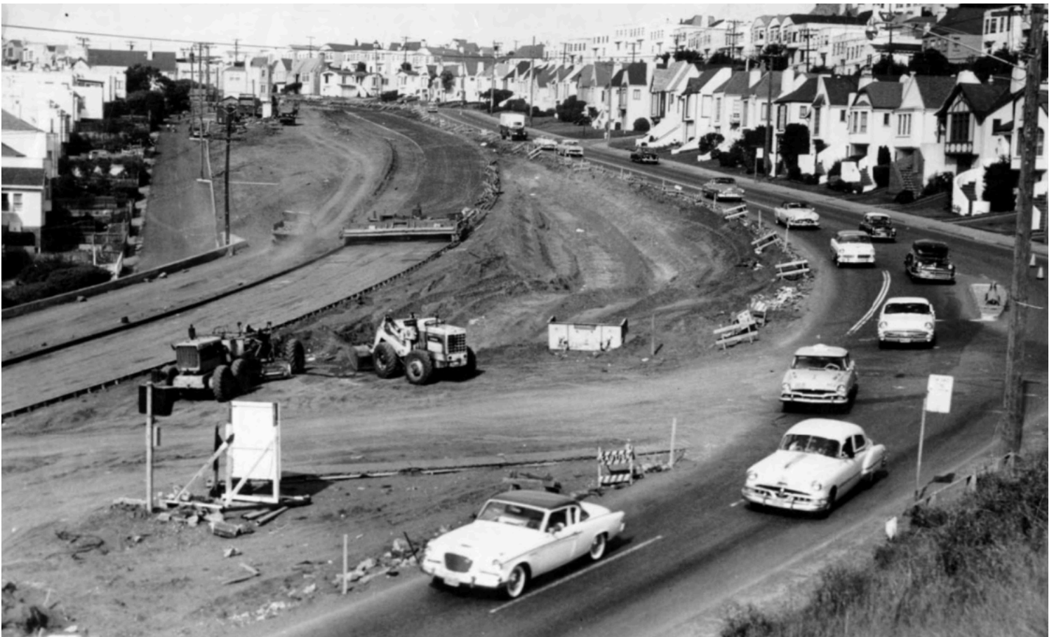
(below) Portola Drive under construction
